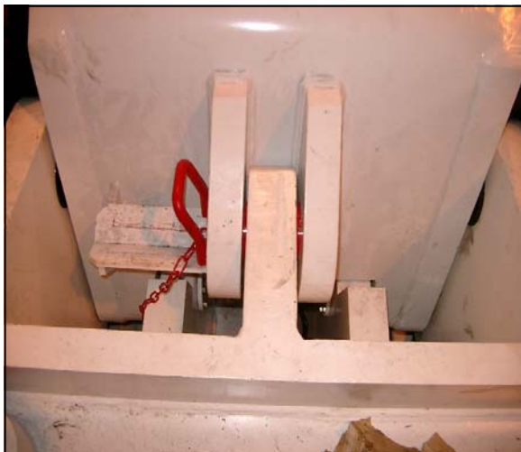
Lift Arm Lock Installed
