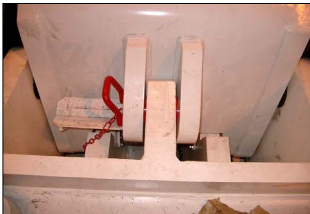
Lift Arm Lock Pin Installed
